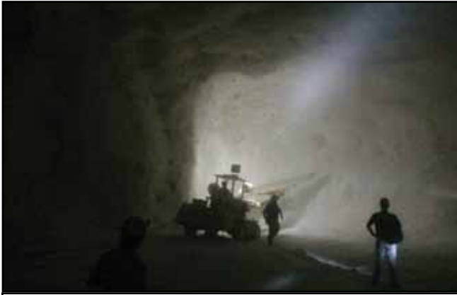
Figure 3: Drilling holes on the salt wall to insert the explosives used in the mining process (E. Kocel photo).
